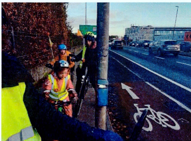
Cyclists wait on narrow footpath to cross N6 to continue inbound trip on inbound cycle track. Headford Road, N6. Desire line now shows majority of cyclists travel inbound on N6 between
