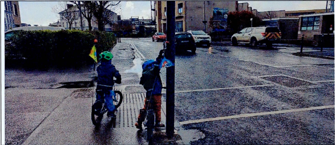
Poor location of toucan activation button – too close to road side.
