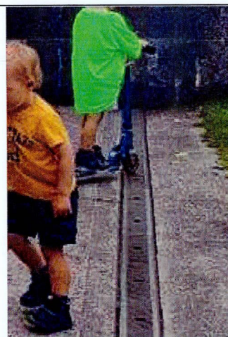
Recessed drainage channel provides safer level surface for pedestrians and cyclists to move across.
