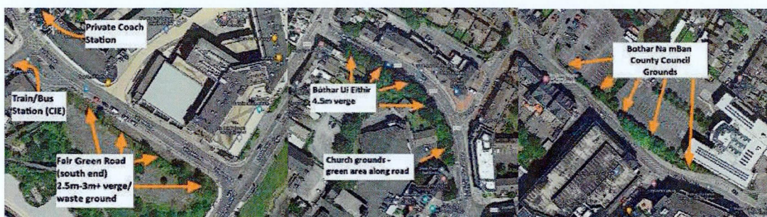
Figure: Captioned Google Satellite View screen grabs of sections from the corridor serving the train and private coach stations, South to North (L to R) Fair Green Road, Bóthar Ui Eithir and Bóthar na mBan. In direct conflict with longstanding state policy, there is no cycling provision directly serving the train station. In all the sections shown there are verges, waste ground or public lands that the designers have made no apparent attempt to use.
