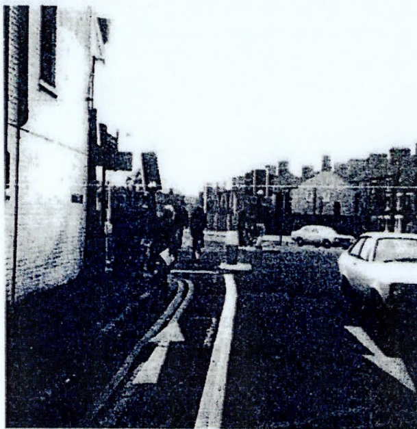
Figure 6: Contra-Flow Cycle Lane and Signal Installation in Peterborough, England
